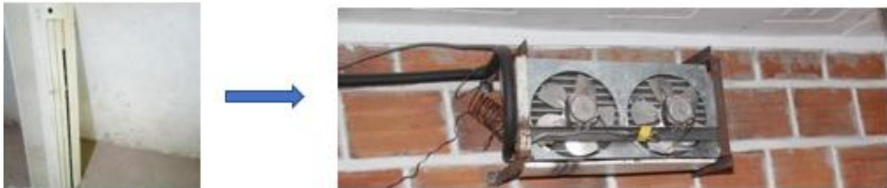
Figure 6-5: Modified Split AC units - locally fabricated fans to blow cool air
