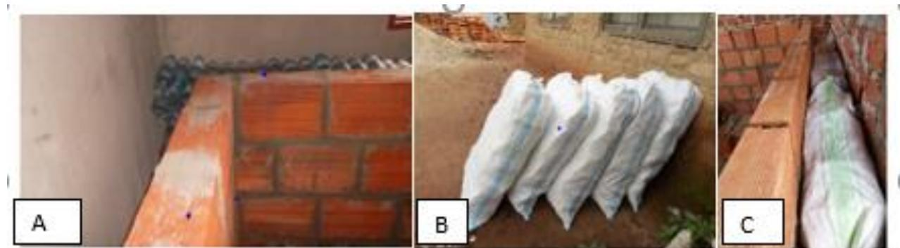
Figure 6-1: **A**- Insulation used in the 1<sup>st</sup> prototype, **B&C**-Insulation board used in second prototype
